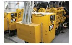
The seismically certified generator sets are mounted on a series of shock absorbing coil springs to minimize vibration. This is helpful in that magnetic resonance imaging (MRI) machines are located in an adjacent building, Schreckengast says.
